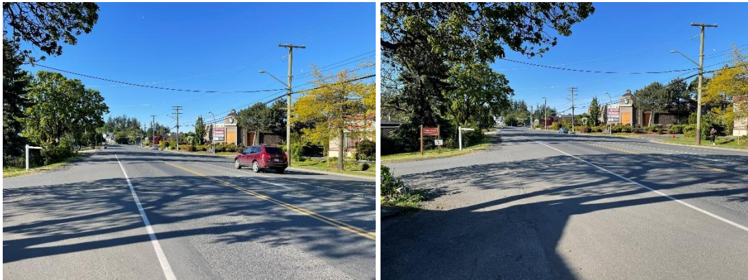
The absence of a sidewalk on the east side of Admirals Road and lack of crossings along the corridor result in a less comfortable and safe experience for people walking.
