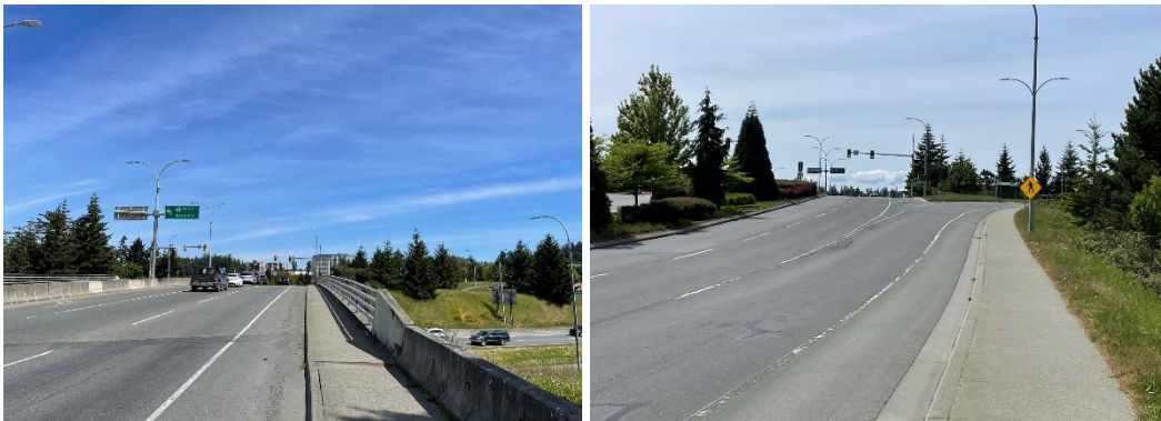
Narrow sidewalk on east side of Helmcken Rd overpass (left). Photo at right is Helmcken Rd looking south. It shows the dangerous transition from the painted bike lane where a person cycling has to cross a busy motor vehicle travel lane.
